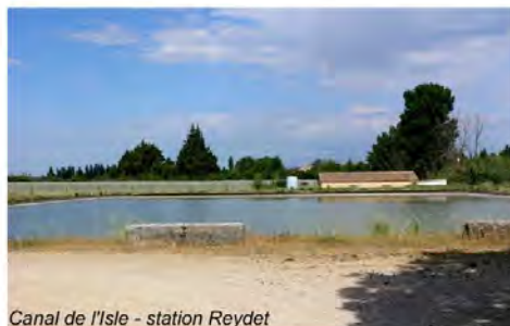
Canal de l'Isle - station Reydet
