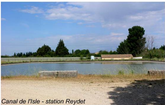
Canal de l'Isle - station Reydet
